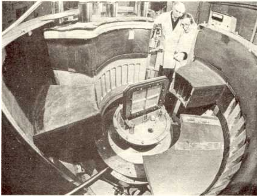
NERA-PR inelastic scattering spectrometer of inverted geometry on beam 7b at the IBR-2 reactor
