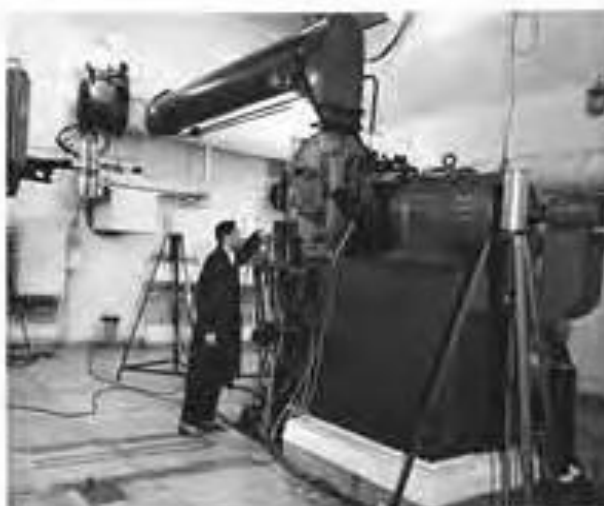
The photo shows the world's first research pulsed fast neutron reactor of periodic operation (IBR).
