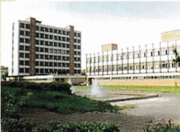
The administrative building
