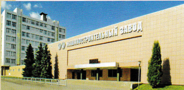
OJSC “Machine-Building Plant” site
